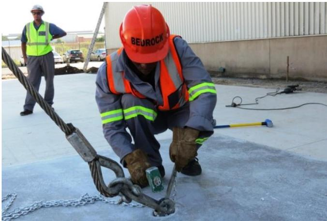
Once the panel is ready to be lifted the crew attaches the quick-release clutches to the lifting inserts.
