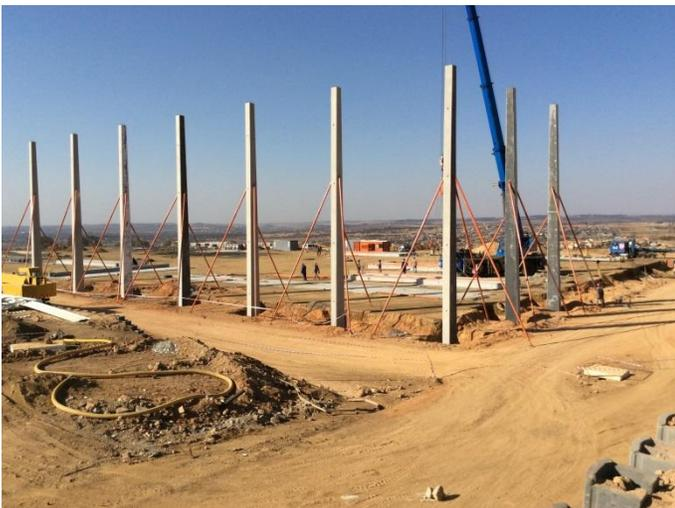
Site-cast is the ideal solution for large concrete columns. Time and cost savings and safety are just some of the advantages over conventional building.
