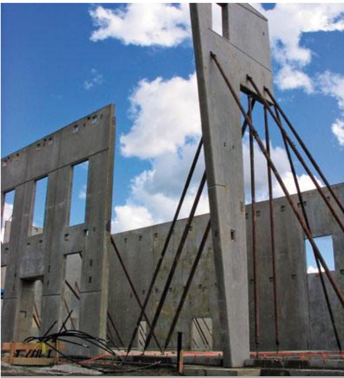
Large complex multi-storey panels positioned and braced.
