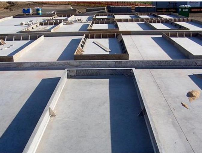
The tilt-up panels are poured into formwork that provides the exact size, shape and openings to meet the design specifications. The largest panel used for a tilt-up construction project weighed over 70T.
