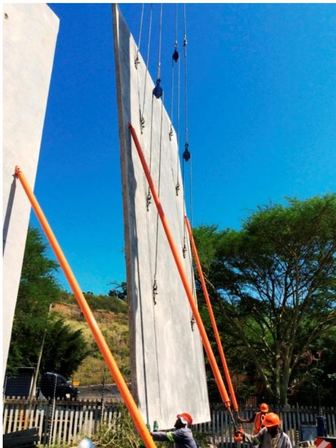
The panel is lifted and tilted into position over the footing by mobile crane. Workers guide the panel and keep the braces from getting tangled in the lines. The process for putting up tilt-up panels goes quickly; an experienced crew, like this Bedrock work crew in Durban can tilt up as many as 30 panels a day.
